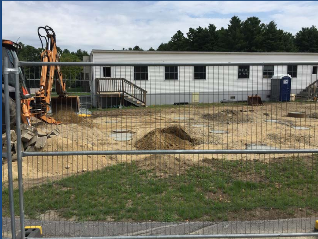
Sanborn Modular Classrooms Installed
