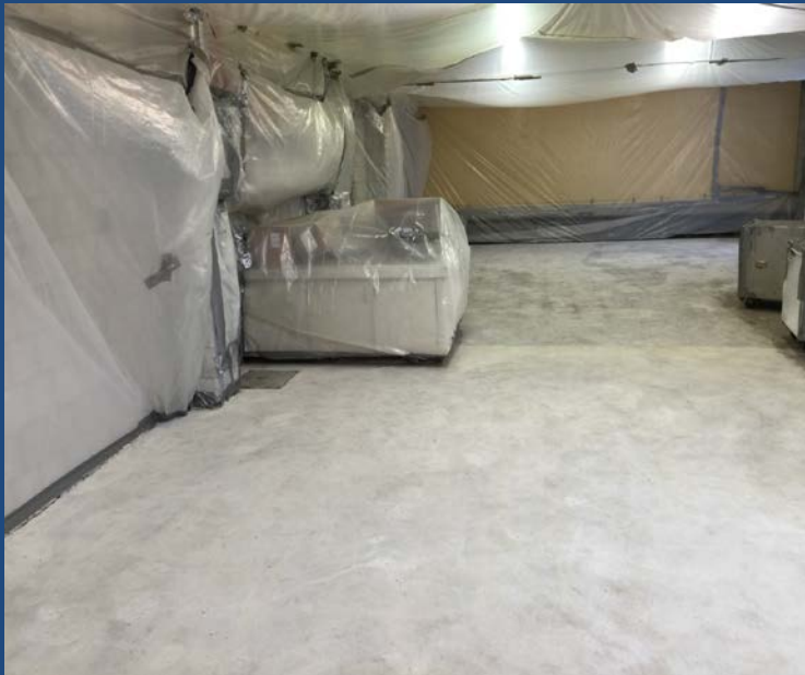
Ripley Copy Center Asbestos Flooring Replacement
