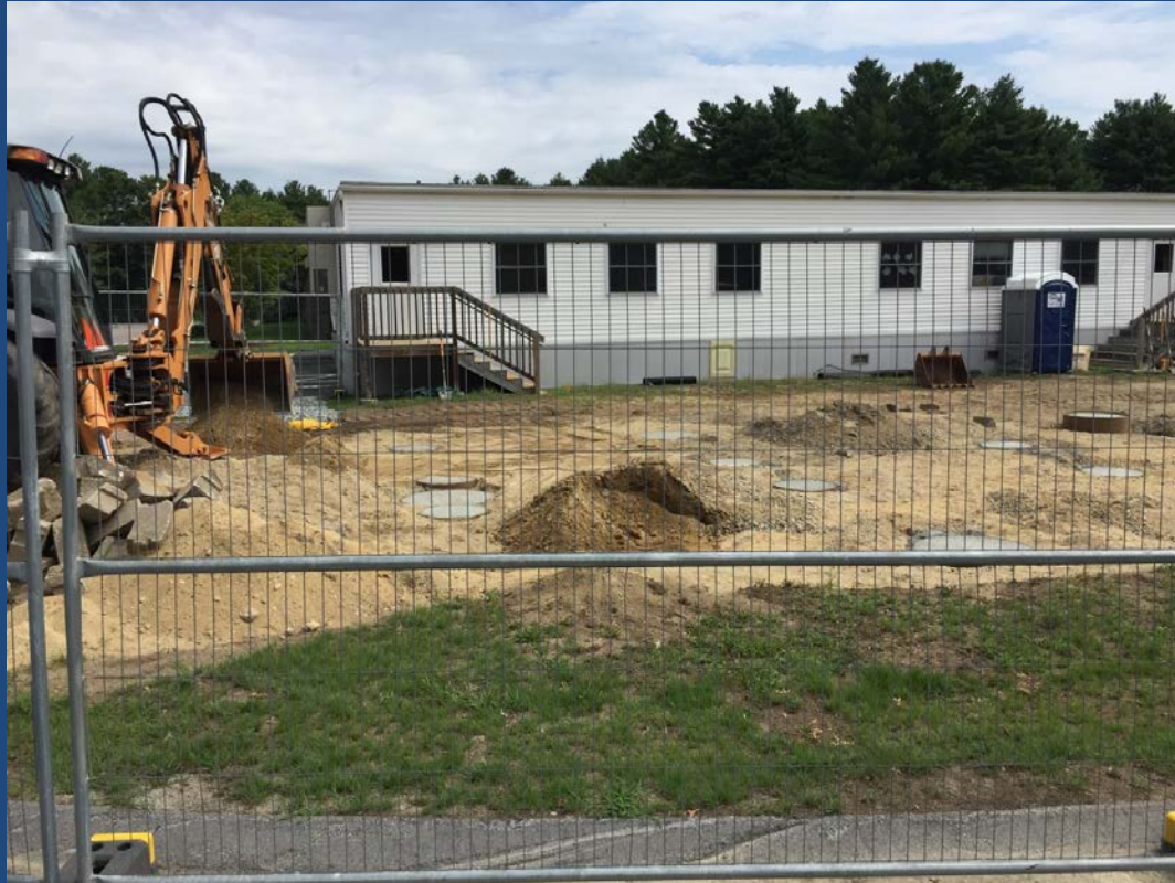
Sanborn Modular Classrooms Installed
