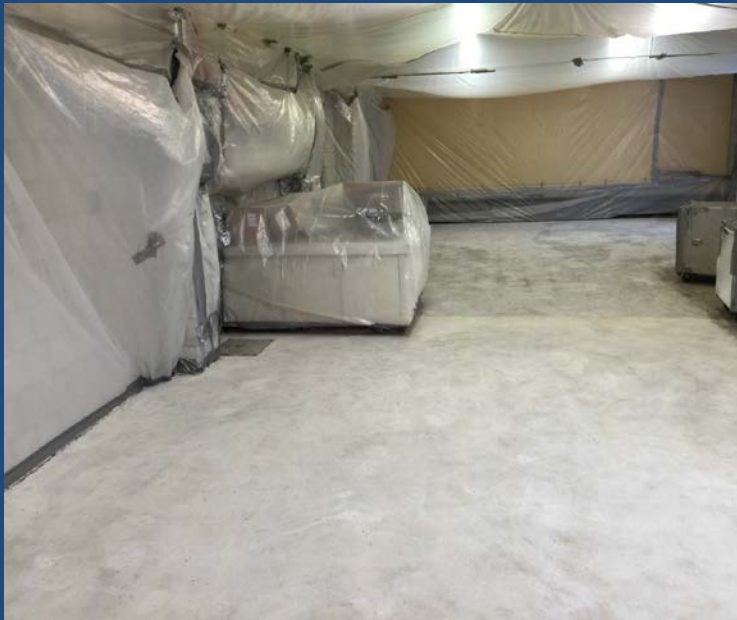
Ripley Copy Center Asbestos Flooring Replacement
